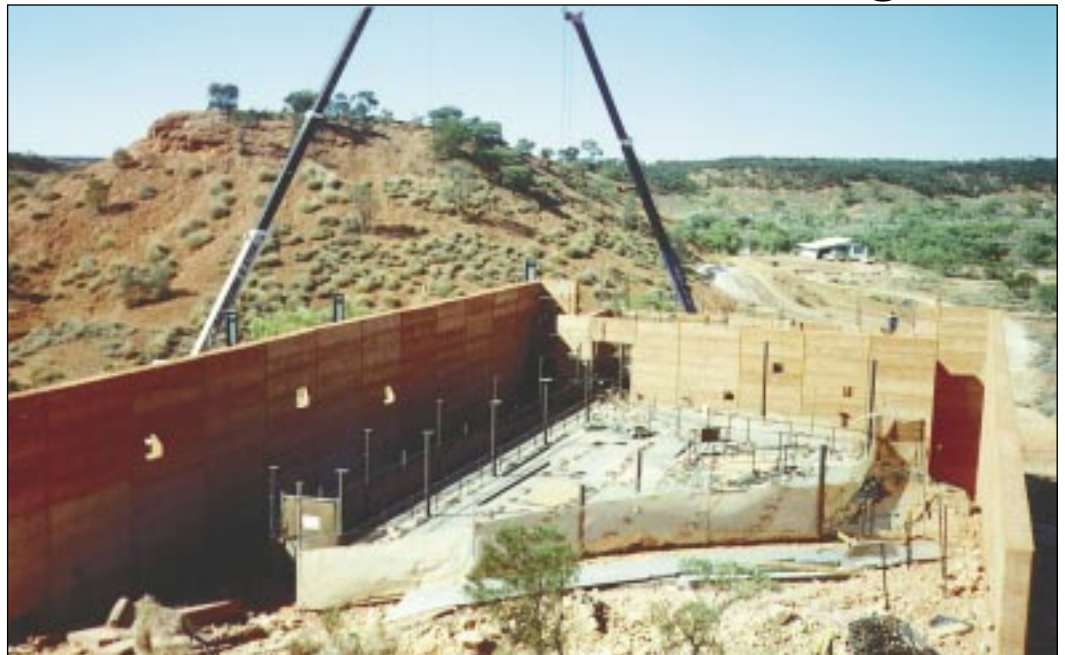
Rammed earth walls were used in construction of the building to house dinosaur tracks.
